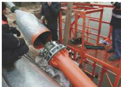
Friction damper installed prior to covering with anti-vandalism protection
